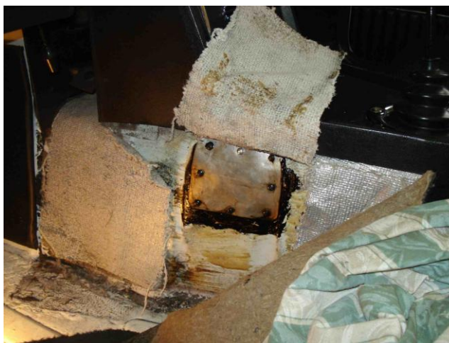
Fig 5. Cover plate fitted.
